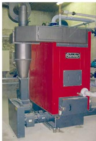
Figure 1-11: Boiler of 130-250 kW capacity (Binder, sold in Austria)
