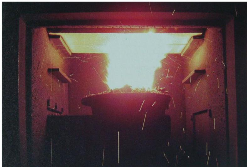
**Figure 3-10: Well controlled combustion in retort boiler**
