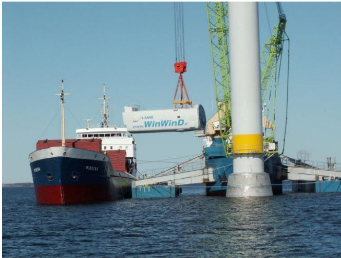
Figur 11.3 Nacellmontage
