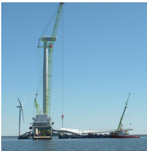
Figur 11.4 Rotormontage
