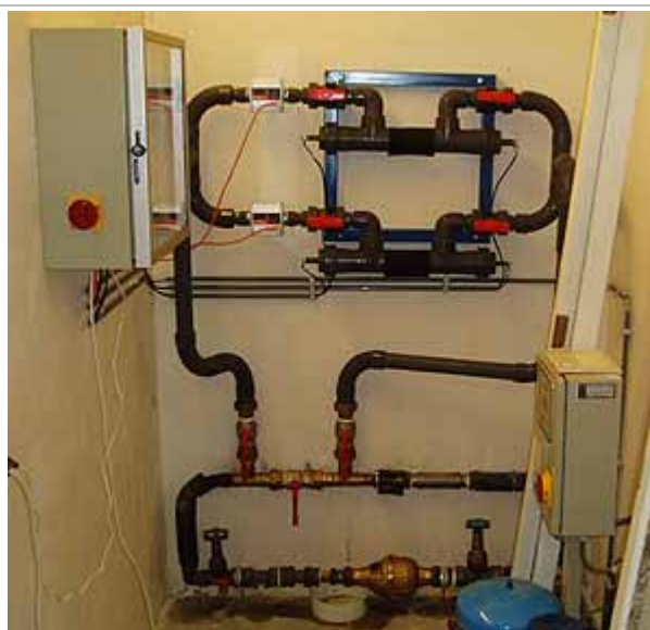
Figure 16-21. Copper-/Silver ionisation system by WTN, Netherlands (Picture: www.waterforum.net)
