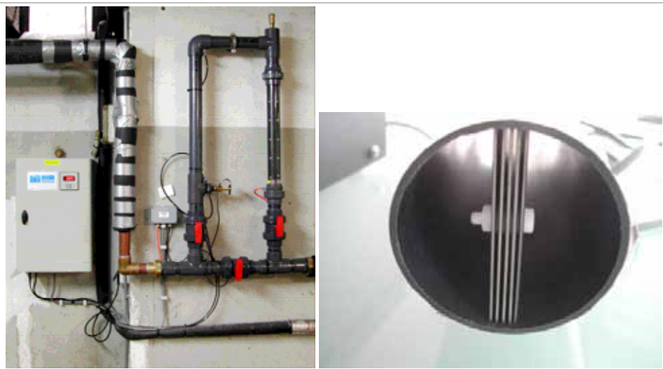
Figure 16-22. (left): Anodic oxidation system (picture: www.brightspark.nl ). Figure 16.23 (right): The electrodes in close-up, placed in a plastic tube segment (picture: www.brightspark.nl )
