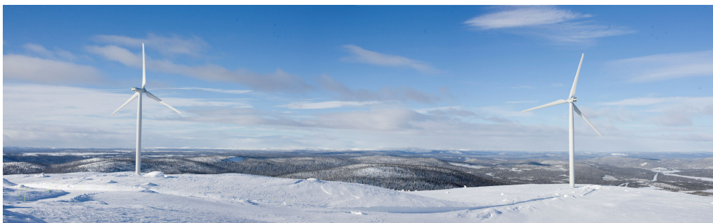
Two of the wind turbines on Uljabuouda
