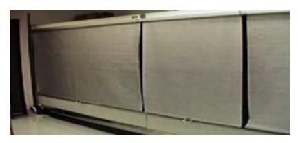
The refrigeration load of supermarkets is reduced by 35 % in summer and 28% in winter when night covers are used for an average of 15.5 hours per day<sup>8</sup>. Many manufacturers claim that night covers can block up to 70 % of the ambient heat that normally enters the cabinet. Night covers can also be used for cabinets with glass doors to improve the insulation.
