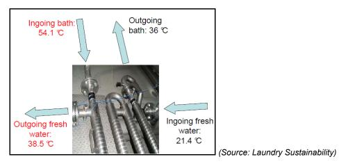
Figure 3 Corrugated pipe heat exchanger of Kannegiesser
