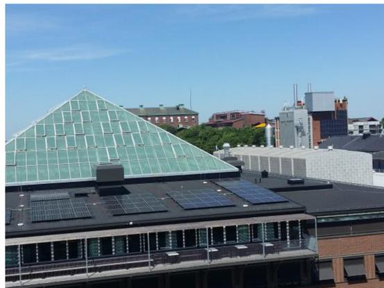
Figure 2 : Solar panels mounted on the roof of the Architecture building and on the wall of the building, where the CHP plant is located.
