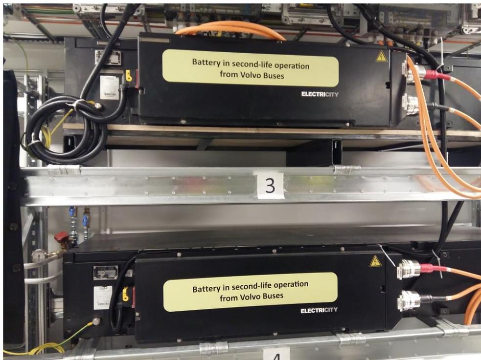
Figure 7 : Second life Li-ion batteries of Brf Viva.
