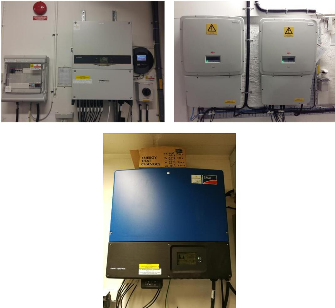
Figure 3 : PV inverters at Chalmers.
