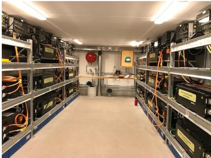
Figure 6 : The second life Li-ion batteries of Brf Viva.
