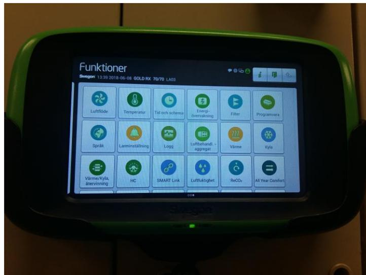
Figure 5: The graphical interface and the functionalities of a building controller located at one of the buildings on Chalmers campus.
