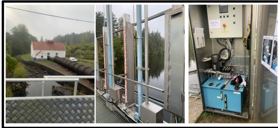
Hydraulic system for water outlet
