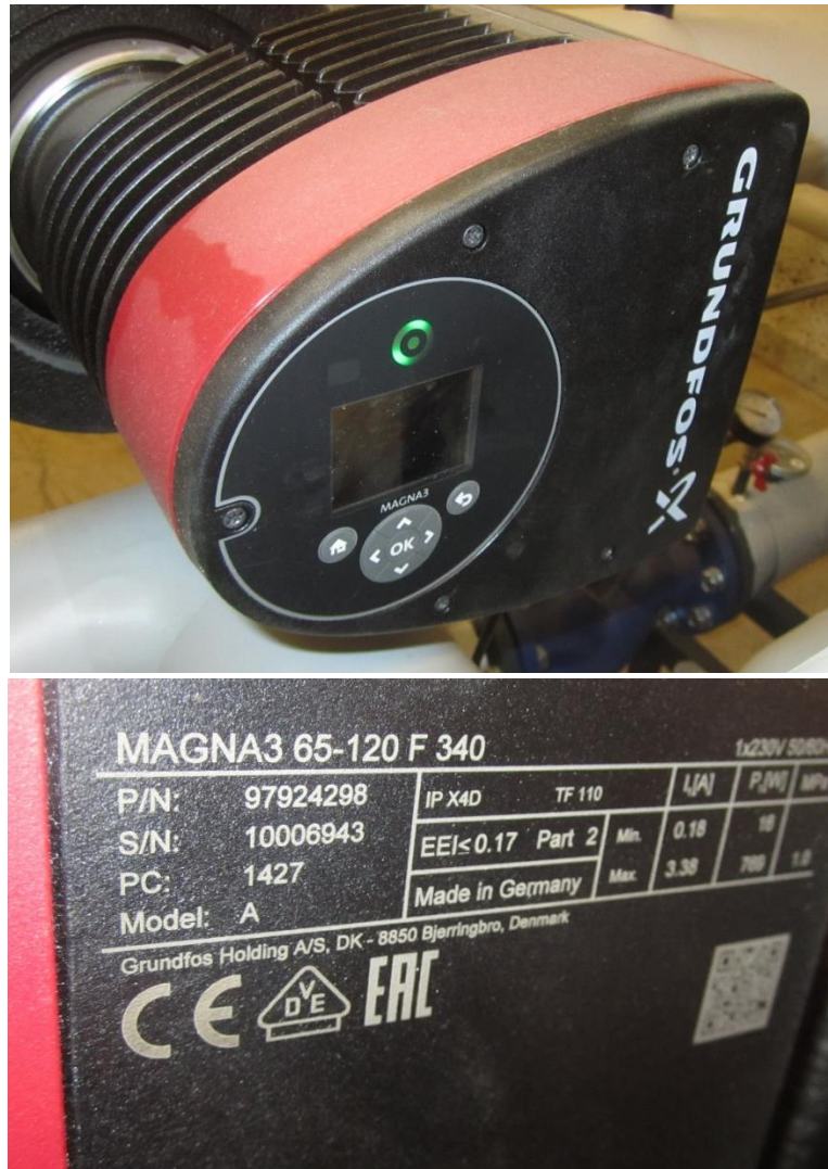
Figure 10: Example of a modern high energy efficient circulator with an EEI of less than 0.17 - top front view of the circulator, bottom side view of the circulator with the name plate showing the EEI.
