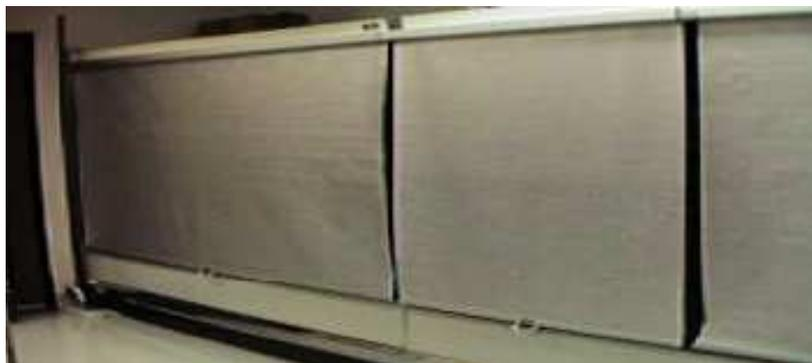
The refrigeration load of supermarkets is reduced by 35 % in summer and 28% in winter when night covers are used for an average of 15.5 hours per day<sup>8</sup>. Many manufacturers claim that night covers can block up to 70 % of the ambient heat that normally enters the cabinet. Night covers can also be used for cabinets with glass doors to improve the insulation.
