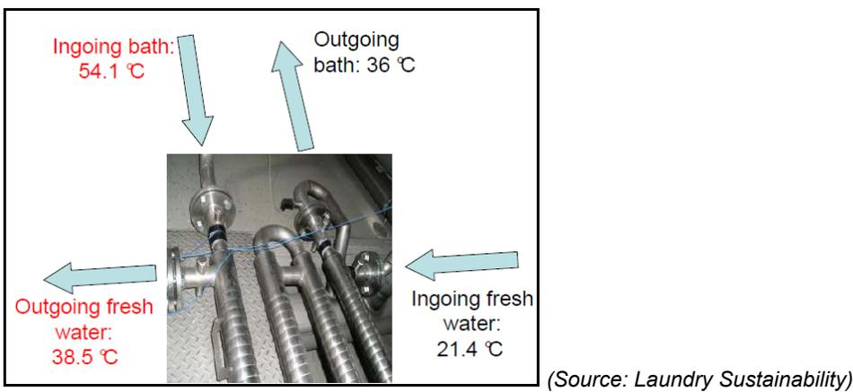
Figure 3 Corrugated pipe heat exchanger of Kannegiesser
