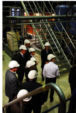
Study visit at the district cooling plant.
